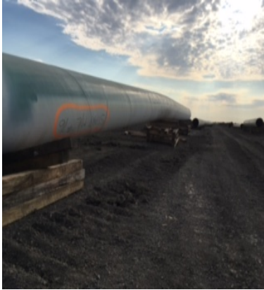
Pipe down the Right of way.
